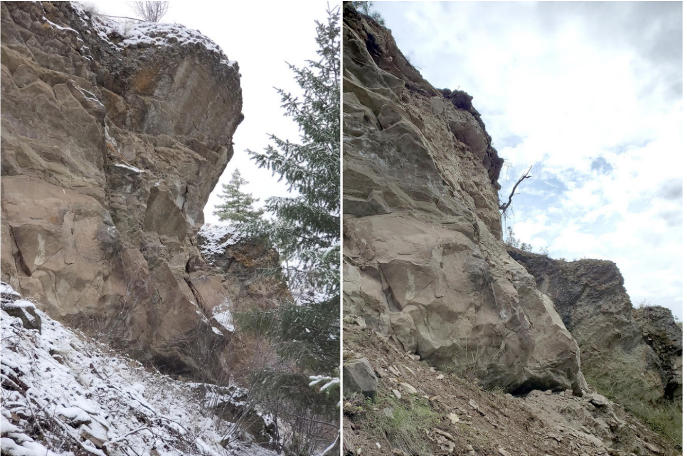
Figure 2: Before and after view of overhanging rock removed by a trim blast (trees along the crest also removed).
