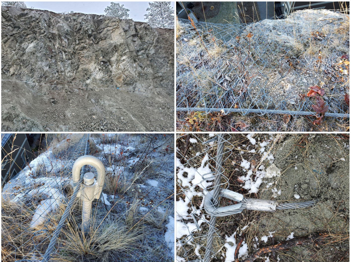
Figure 5: High tensile strength wire mesh draped over a rock face and held by an upper wire rope; different techniques are used to anchor the wire rope and keep the wire mesh drapery close to the rock surface.
