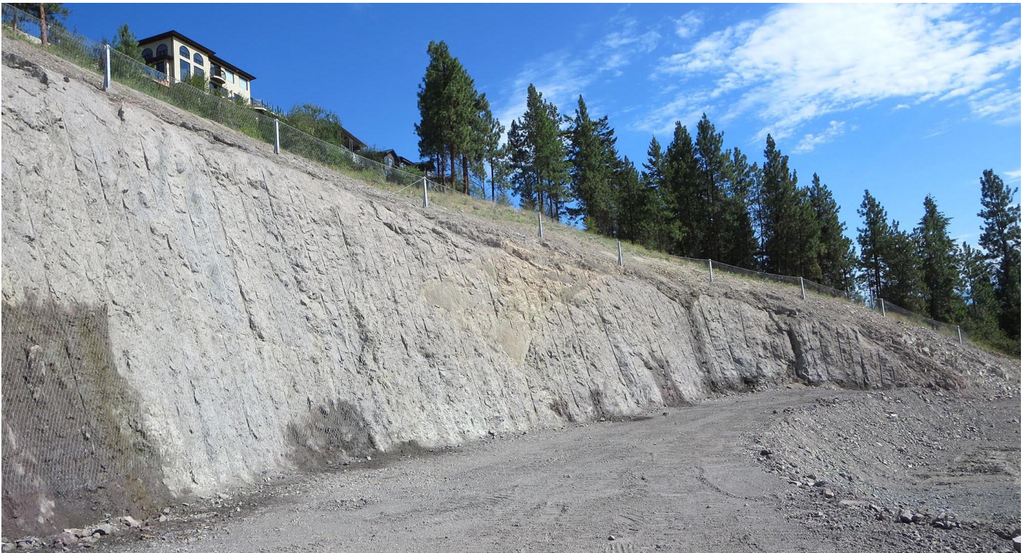
Figure 3: Backyard rock cut implementing multiple rockfall mitigation solutions starting with pre-split blasting.
