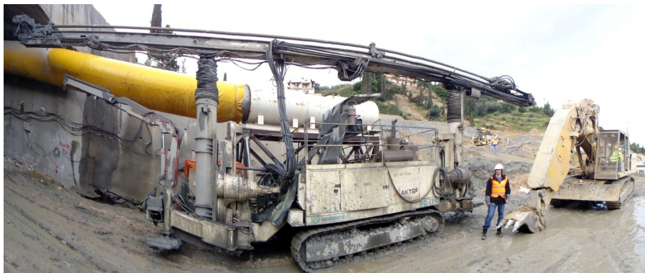
Figure 2 - Case-drilling machine for installing forepole members in the Athens-Patras Motorway, (near Patras) Greece
