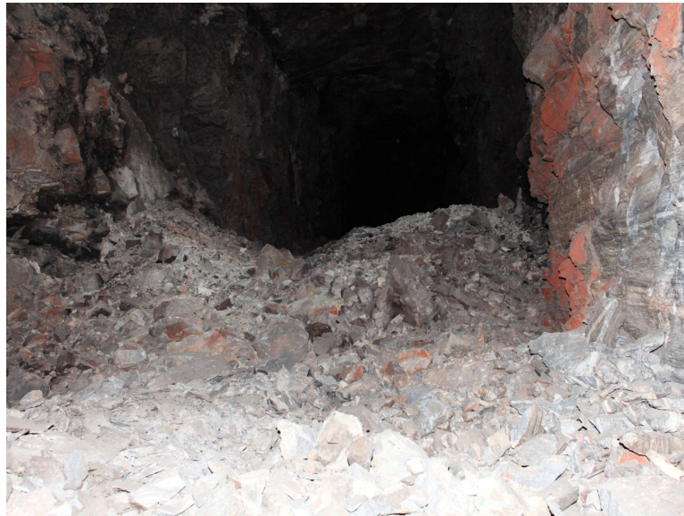
Figure 6 - Severe tunnel damage with spalled rock piled up to 1.7 m deep on the tunnel floor
