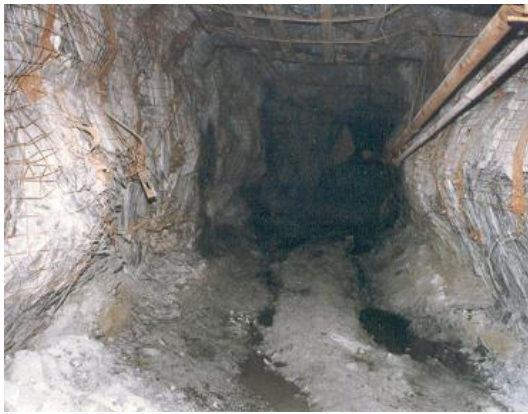
Figure 1 - Squeezing ground conditions
