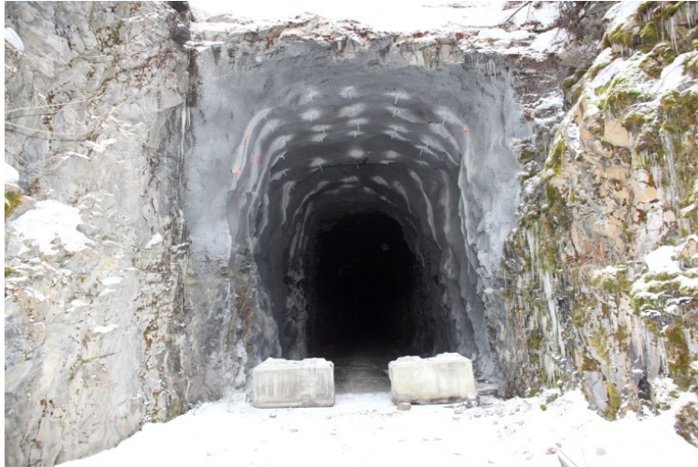
Figure 7 - Northeast tunnel portal showing addition of shotcrete and bolts
