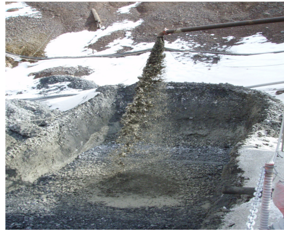
Figure 10 - A CRF preparation pit
