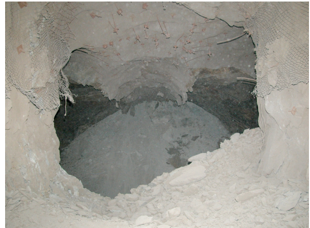
Figure 6 - CRF failed into a lower level stope
