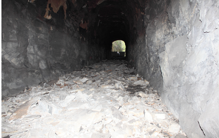
Figure 4 - Rock that has fallen from the roof in the first 80 m of the tunnel
