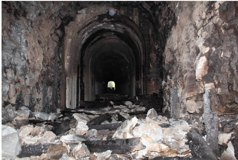
Figure 5 - Concrete arch and severe damage to the rock (110 to 130 m from the portal)
