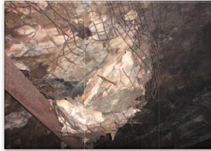
Figure 1 - Ground fall after a seismic event where rock support was corroded
