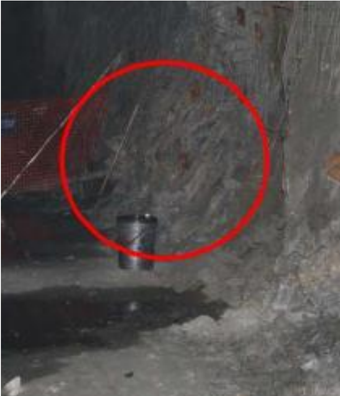
Figure 7 - State of ground support (D-Bolt and mesh) after a 1.9 Mn seismic event
