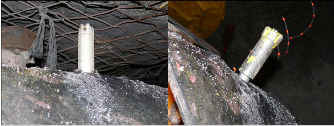
Figure 7 - Drill the rebar hole with different size bits to create a shelter for the U-cell
