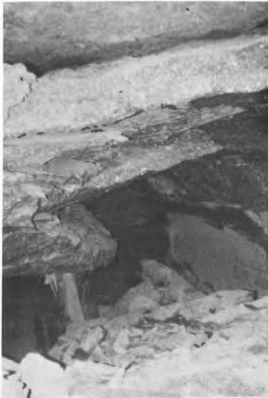
Figure 1a. Massive roof failure of Saskatchewan potash mine threatening safety and economical operation of mine.
