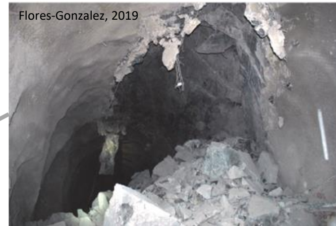
Spalling of extraction level related to locally weak rock in abutment stress zone
